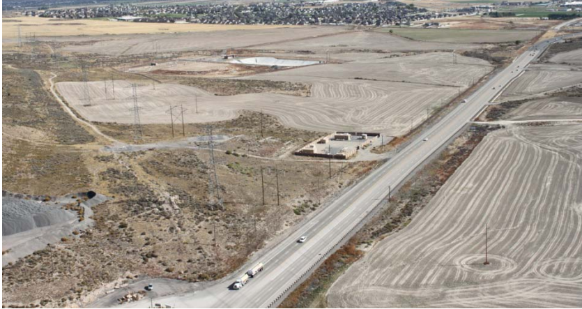
Figure 21: Utility Corridor Crossing at SR-73
